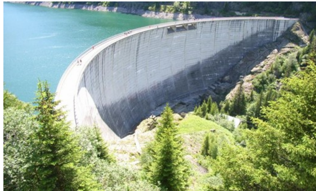
Fig. 1 – Double curvature, 69 m high and 250 m long arch dam in Saint Guérin
