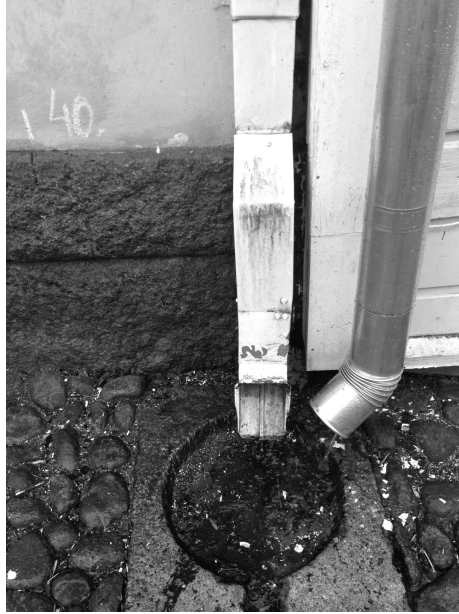
Figure 3. Changes in the sound of rain: older rectangular and newer round and smooth eaves troughs in Piispankatu, Turku. Picture: Meri Kytö
