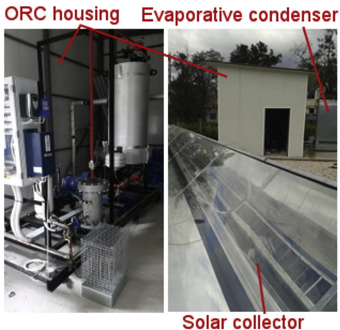
Fig. 3. Solar field and ORC in the housing at the AUA campus.
