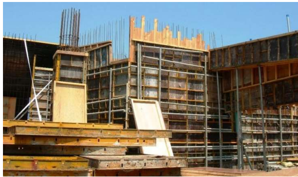
Figure 2: Larch boards mounted on Euro-Form panels
