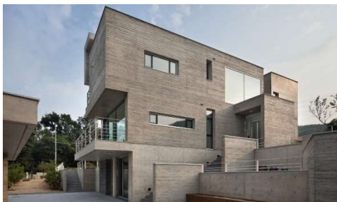
Figure 3 A single family house with two different exposed concrete textures
