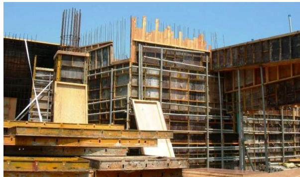
Figure 2: Larch boards mounted on Euro-Form panels
