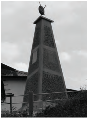
Figure 4-9: A recent pillar at Umden market Ri bhoi district
