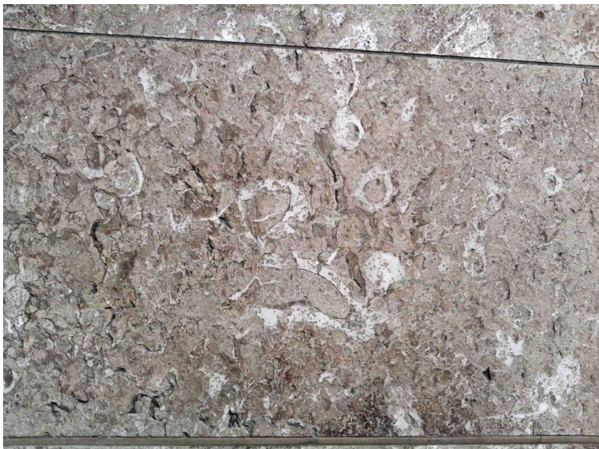
Fig. 13. Paving slabs in Aix-en-Provence TGV station – a local Cretaceous rudist limestone (the rudists are 5-10 cm long) © P. De Wever
