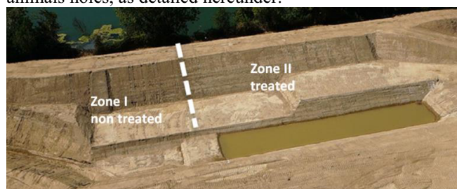
Figure 4. The dike before testing: non treated on the left side, lime treated on the right side
