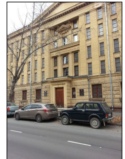
The building of the former Special Archives, now a part of the Russian State Military Archive (photograph taken by Andrei Zamoiski, October 2014).
