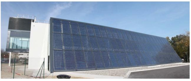
Fig. 1. The Georges Giralt Building: The Photovoltaic Main Windowed Façade
