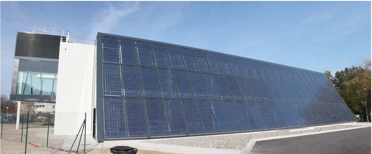
Fig. 1. The Georges Giralt Building: The Photovoltaic Main Windowed Façade
