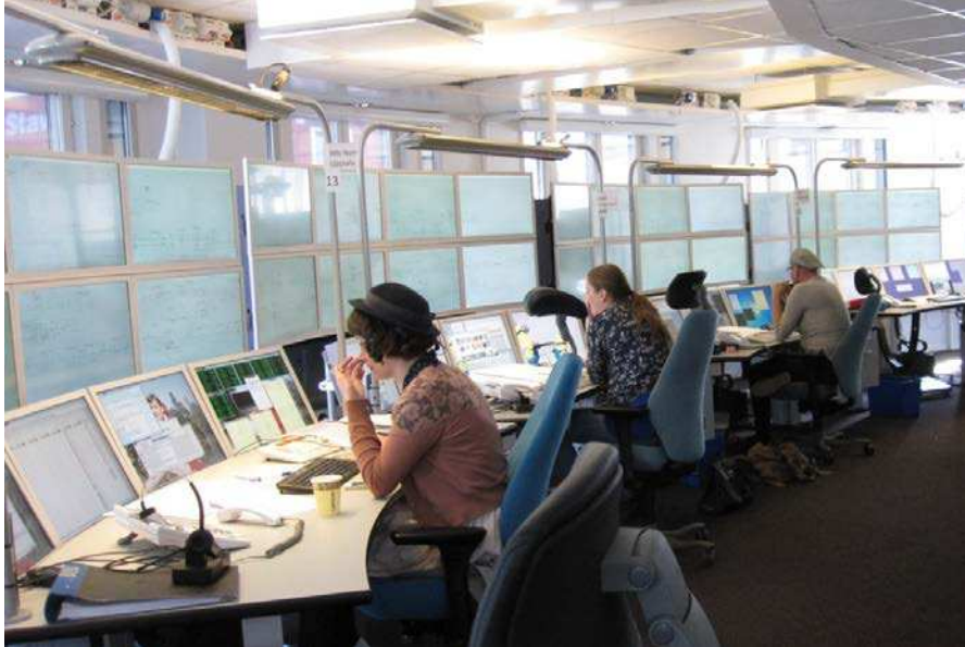
Fig. 2. The same control centre as in Figure 3, but here re-designed for visualization using a number of large size screens at each individual workplace.
