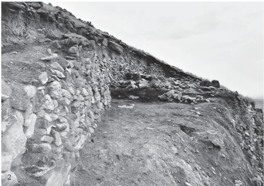
Fig. 23. Chobareti, Lower Operation, Structure 4. 1 Looking north; 2 Looking east.
