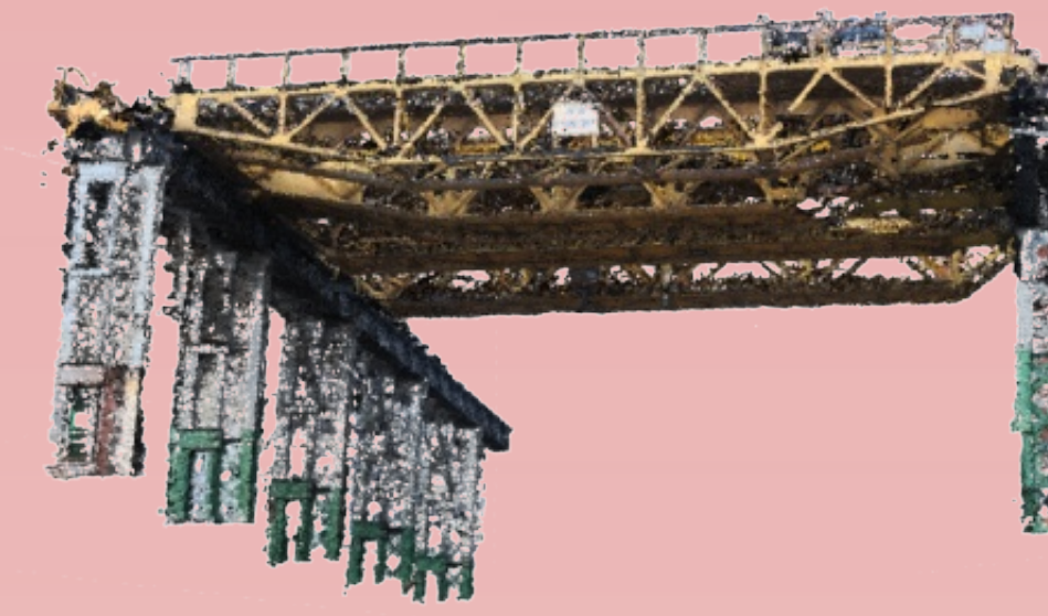
Halles Alstom's Overhead crane
