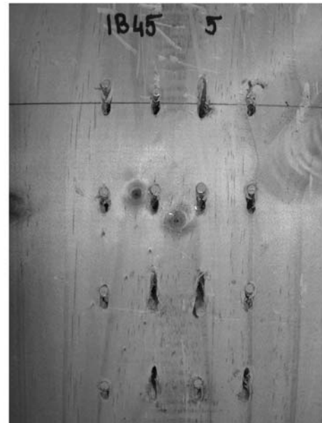
Figure 18: (a) Nails starting to bend and (b) embedment of the nails into the timber (not at scale).
