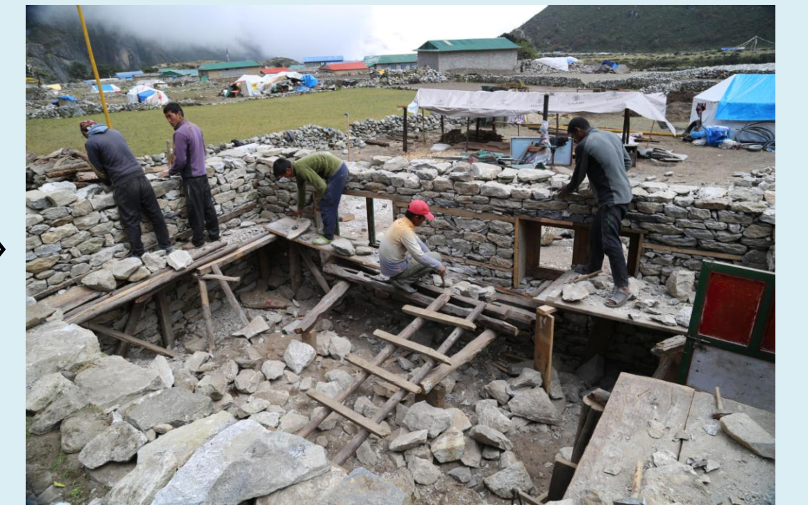
Traditional construction methods throughout many parts of the Himalaya have utilized hand-cut stone blocks with wood spacers, called “timber bands” or “tie beams.” Timber bands tend to isolate smaller portions of a stone wall relative to seismic shaking, thus preventing the entire wall from undergoing catastrophic failure. Timber bands, carved into decorative snakes, are clearly seen in Kathmandu on Hanuman Dhoka Palace (yellow arrows in photo below) in Durbar Square. The old palace experienced far less damage from the Gorkha earthquake than did the newer addition to the palace (white building to the left).
