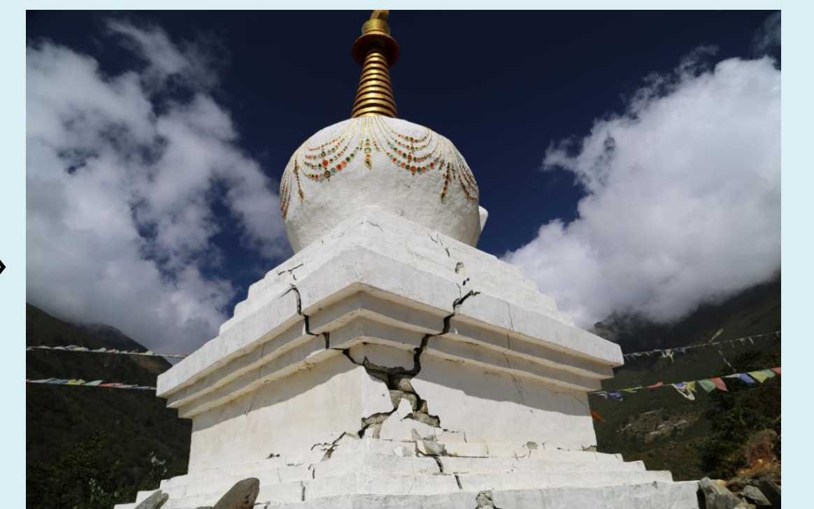
“X-cracking” of external structural walls was common damage from the Gorkha earthquake, often with cracks originating from corners of windows and door jams. Large, through-going sub-vertical cracks were also common, along with topping of stones at the top of walls and from triangular spaces directly under roofs. The Buddhist stupa above, just west of Namche Bazaar, shows a dramatic example of x-cracking at a corner.
