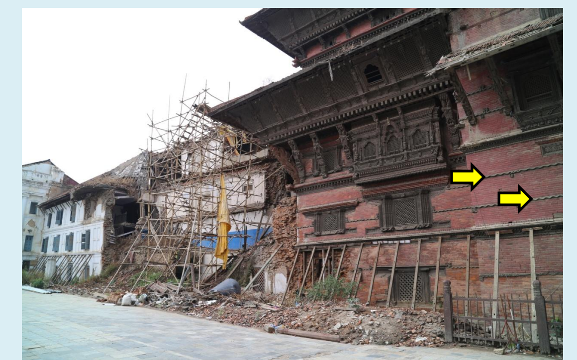
Traditional construction methods throughout many parts of the Himalaya have utilized hand-cut stone blocks with wood spacers, called “timber bands” or “tie beams.” Timber bands tend to isolate smaller portions of a stone wall relative to seismic shaking, thus preventing the entire wall from undergoing catastrophic failure. Timber bands, carved into decorative snakes, are clearly seen in Kathmandu on Hanuman Dhoka Palace (yellow arrows in photo below) in Durbar Square. The old palace experienced far less damage from the Gorkha earthquake than did the newer addition to the palace (white building to the left).
