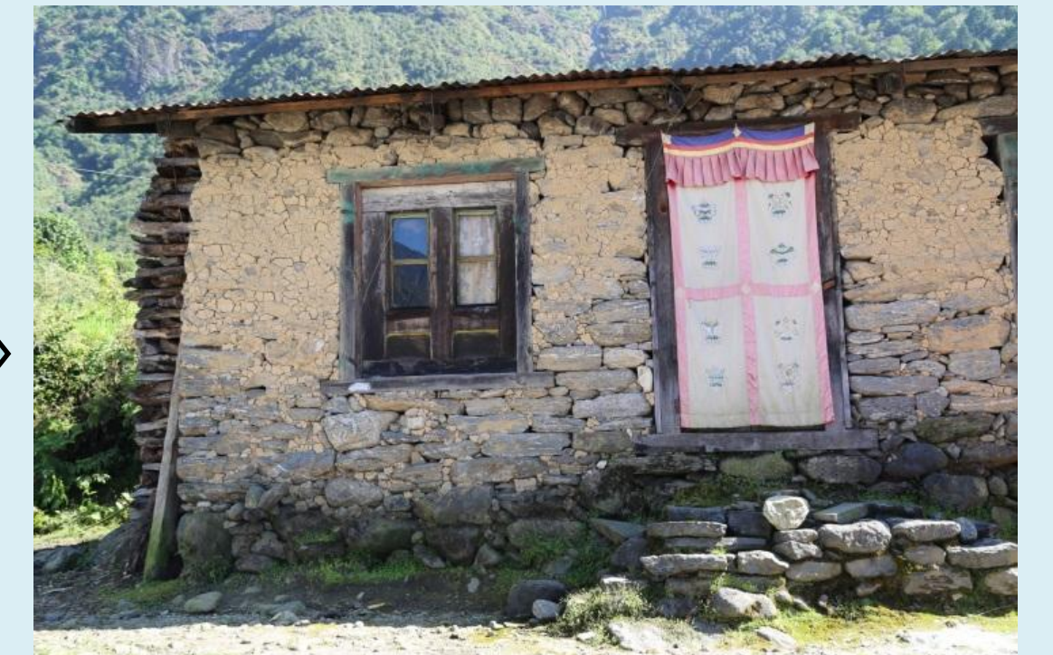
Older, traditional buildings in the Khumbu were constructed of uncut “field stone” with no mortar or external plaster, just small stones placed between larger stone blocks to fill gaps; some buildings used dried mud mortar as an external “plaster”, as shown in the diagram and photo above (Lukla).
