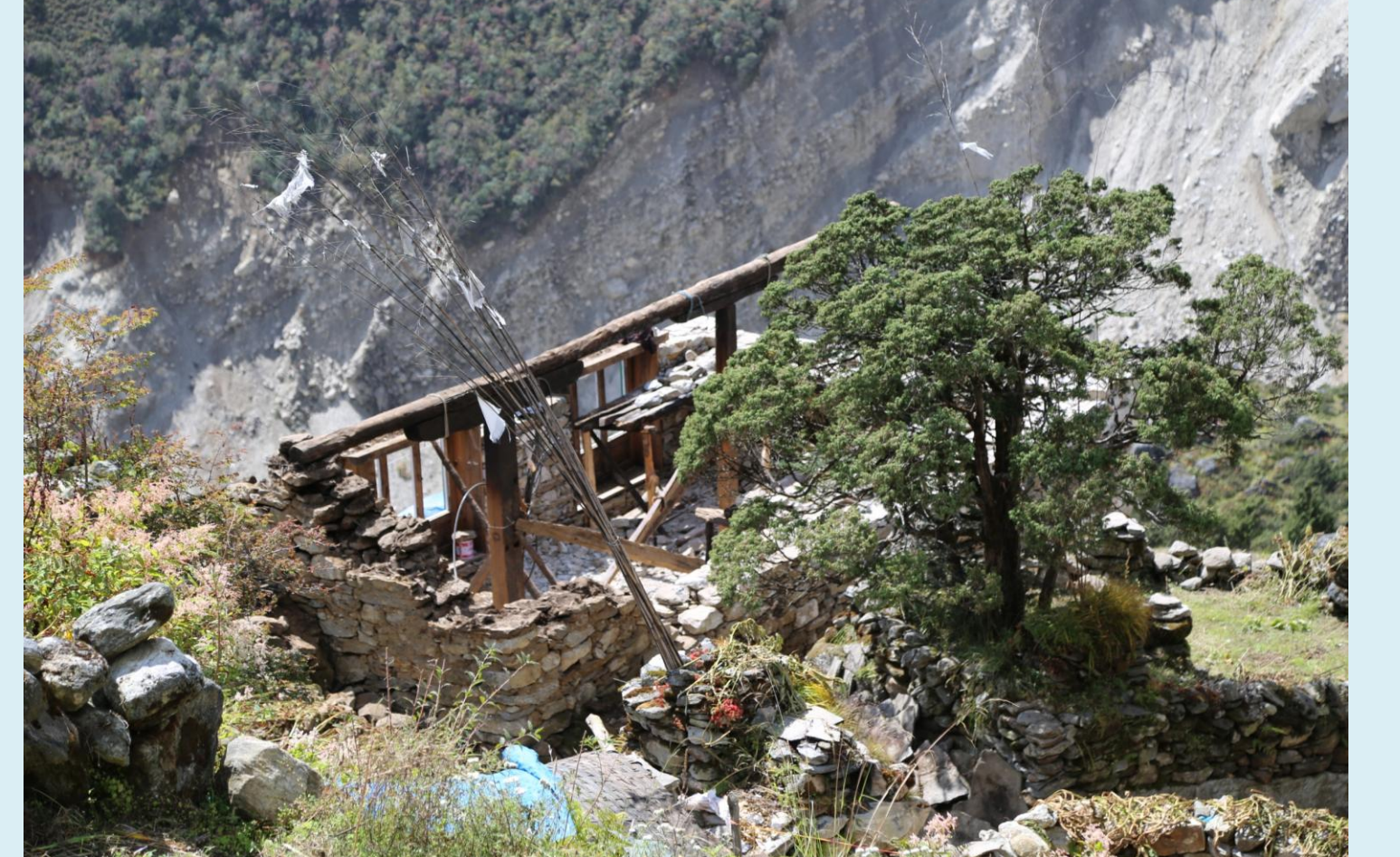
ABOVE: Catastrophic failure of roof and walls of a traditional Khumbu building (stacked field stone with external plaster) near Thame. BELOW: Thame experienced massive damage during the Gorkha earthquake and its aftershock sequence; this famous Sherpa village was constructed on water-saturated ground moraine and outwash between high lateral moraines. Many people still live in make-shift shelters of tarps, sheet metal, or whatever else can be salvaged.
