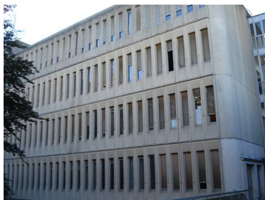
Figure 8: IT A Building.
