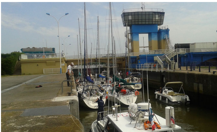
Fig. 6.6 The lock of the Arzal dam (Source IAV, with authorization)
