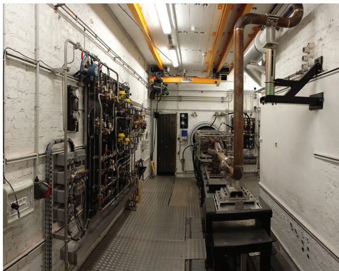
Figure 20 – The MICADO test rig under development
