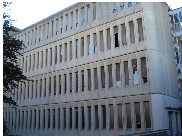
Fig.1. Building A of the Telecom SudParis Institute
