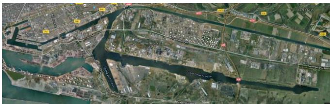
Fig. 2: Aerial view of the French port industrial zone of Le Havre (Google Maps)
