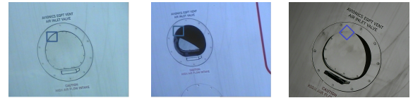
Figure 9: Air inlet vent - sliding window inspection.
