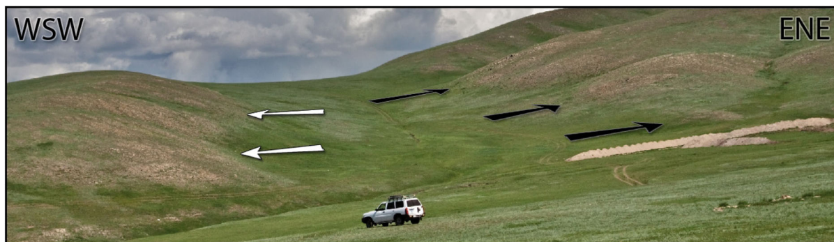
Figure 3. Picture of the survey area (see Fig. 2 for location). Black arrows highlight the Emeelt fault scarp and white arrows show another morphological scarp. The trenches are visible on the right side.
