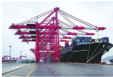
Fig. 1 the photo of Ship-To-Shore quay-side container cranes (STS)
