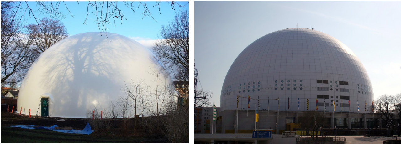
(a) Air inflated structure in Gentofte (Denmark) 1 . (b) Stockholm Globe Arena (by Tage Olsin CC BY-SA 2.0).
