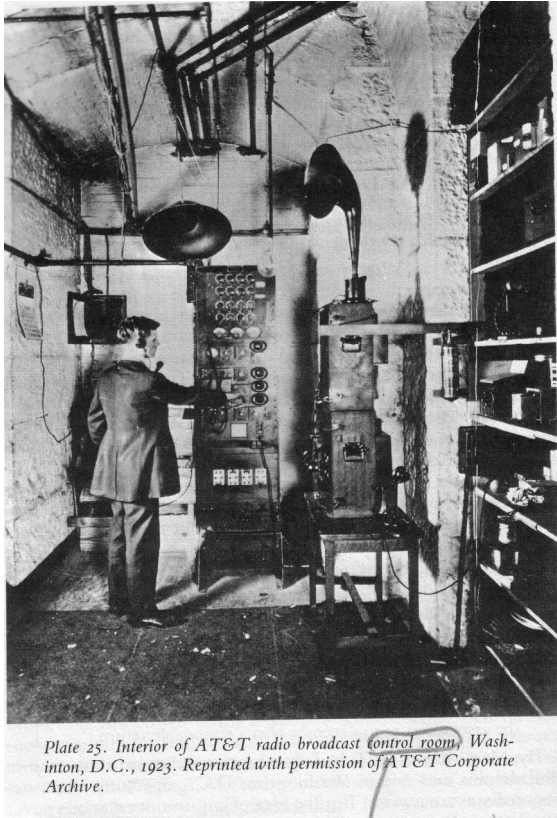
Figure 4 AT&T Control Room, 1923
