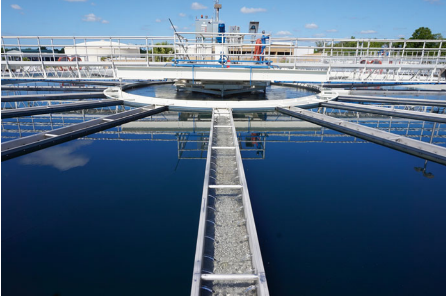
Fig. 2.2 Peace River Manasota Regional Water Supply Authority Water Treatment Plant facility. Water decontamination corresponds to one of the several regulatory costs induced by pesticide use. Estimates of regulatory costs differed considerably between studies, depending, in particular, on whether or not they considered the control of underground water. For instance, in the United States, Pimentel and coworkers began to consider the costs of monitoring underground water and wells in their papers published in 1991. The consideration of these costs led to an immediate increase in their estimates of the overall cost of pesticide regulations of more than 300 %, with these costs accounting for 90 % of total regulatory costs for pesticide use (Pimentel et al. 1991a, b). Moreover Pimentel (2005, 2009) and Pimentel and Burgess (2014) estimated that the current monitoring of wells in the United States (about US$2 billion per year) would have reached US$17 billion per year if all the wells in the United States were monitored (Unmodified photography by Florida Water Daily, under Creative Common License CC BY ( https://creativecommons.org/licenses/by/2.0/ ))
