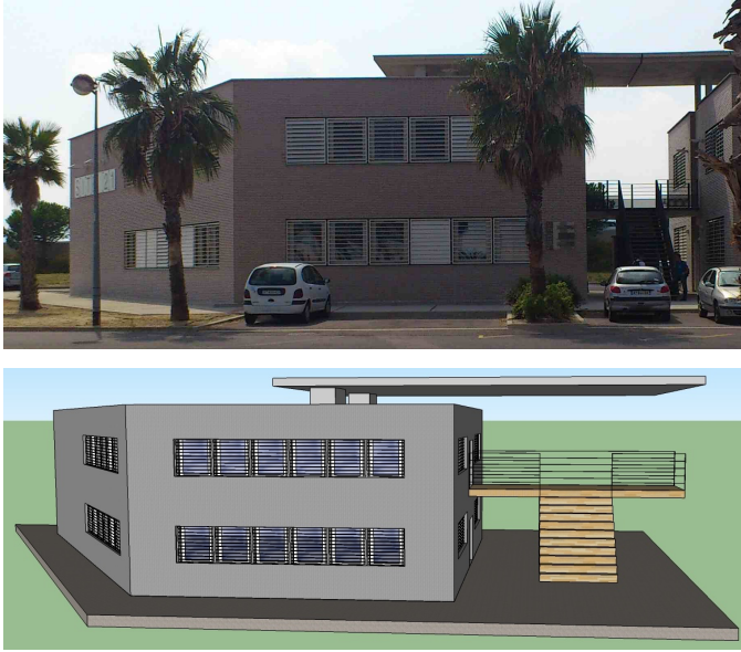
Fig. 1. Photography of the two floors building under study and the corresponding Google Sketchup mock-up.
