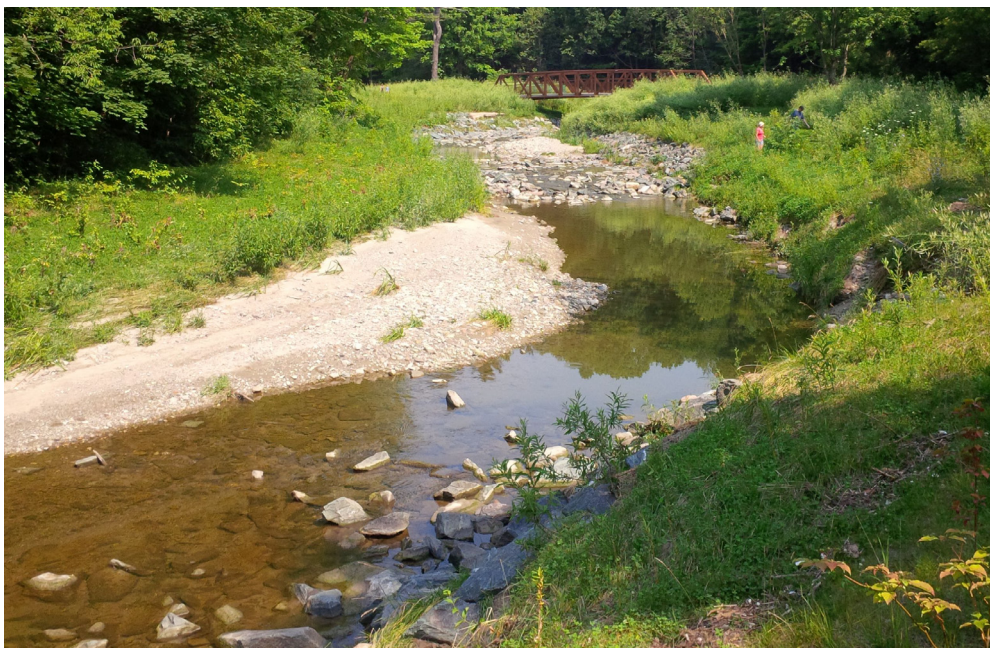
Figure 3. Photograph of restoration site July 2013, approximately 18 months after construction. Note the rocky riffle upstream of the pool in the middle of the frame and the point bar largely formed from deposited sand and gravel. Flow is from top to bottom.
