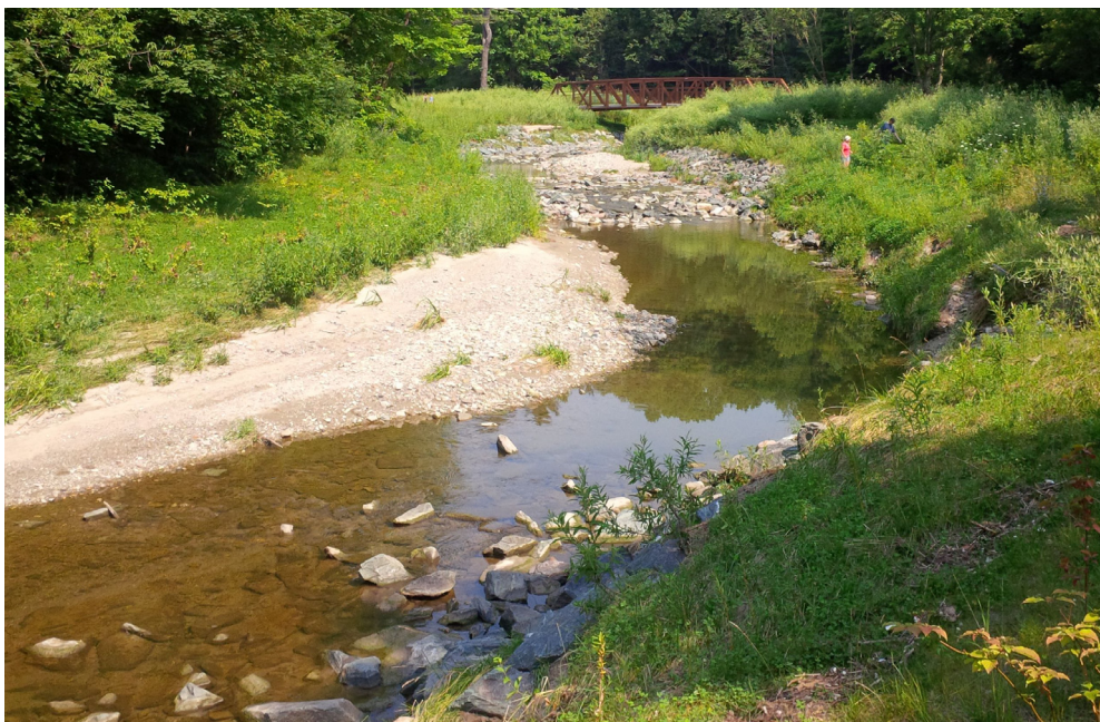
Figure 3. Photograph of restoration site July 2013, approximately 18 months after construction. Note the rocky riffle upstream of the pool in the middle of the frame and the point bar largely formed from deposited sand and gravel. Flow is from top to bottom.
