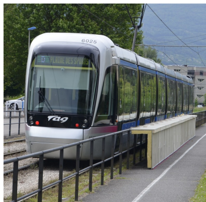
Figure 3: View of the noise barrier prototype with a Alstom Citadis 402 tramway of the Grenoble B line passing-by. The length of the barrier is about 22 m, whereas the tram is about 43 m long.
