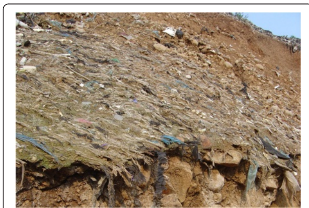
Figure 7 Pieces of plastic bags displaying horizontal orientations along the post-disaster scarp of the dump (Photo: F. Lavigne, July 2005).
