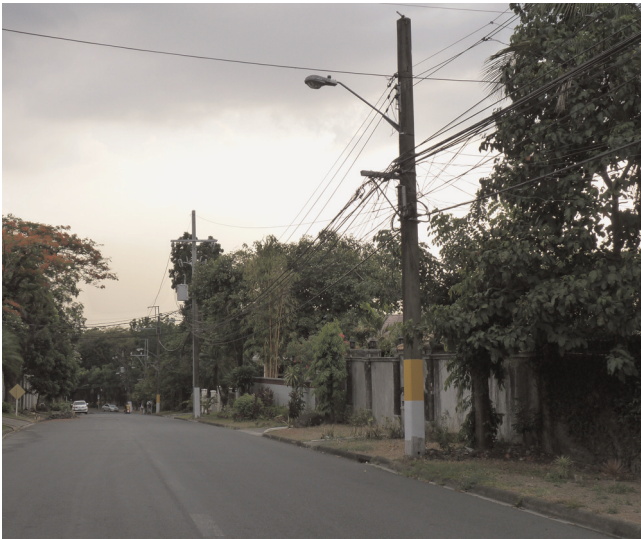
Picture 2. Loyola Grand Villas, Quezon City, Metro Manila, April 2014.
