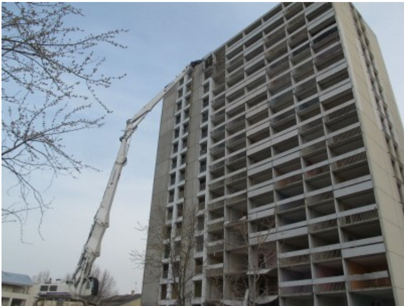
Figure 2- demolition of a tower, District in Romans-sur-Isere , ©Karin SCHAEFFER
