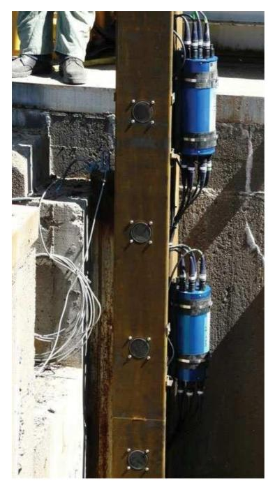
This is a close up of horizontally installed ASFM transducers on a steel frame used for flow measurement.
