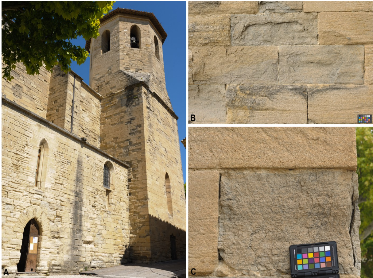
Figure 1. Views of church Saint Maurice of Caromb (14 th century, Vaucluse, France) showing the high degree of spalling decay on the bell tower (A), and the eastern façade (B). The superficial state allows distinguishing a limestone type strongly affected by spalling (grey facies) from one moderately affected (yellow facies). Details highlight the progressive plate formation affecting a grey ashlar viewed from the side (C): the plates vary in thickness and are isolated from the bulk by a fractured zone.
