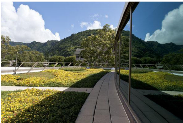
Fig. 1 A 2,500 square foot green roof at the LEED Platinum Laboratory, the Center for Microbial Oceanography: Research and Education, C-MORE Hale, University of Hawaii at Mānoa
