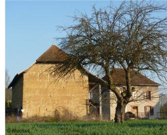
**Rammed earth building** involves compacting layers of earth into a formwork to create walls (pict.2). Widely used in Rhone-Alpes region before it declined after the Second World War, the technique has turned in the last decades to be promoted by a wide range of actors, from architects and researchers to craftsmen, inhabitants, politics or even materials producers.
