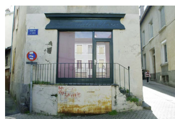
Fig.42 Local commercial vacant
