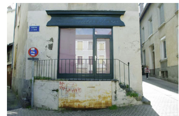
Fig.42 Local commercial vacant
