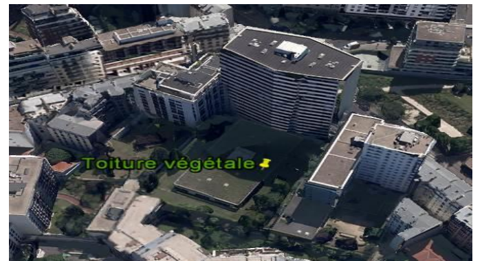
8 - Green roof (15 th )
