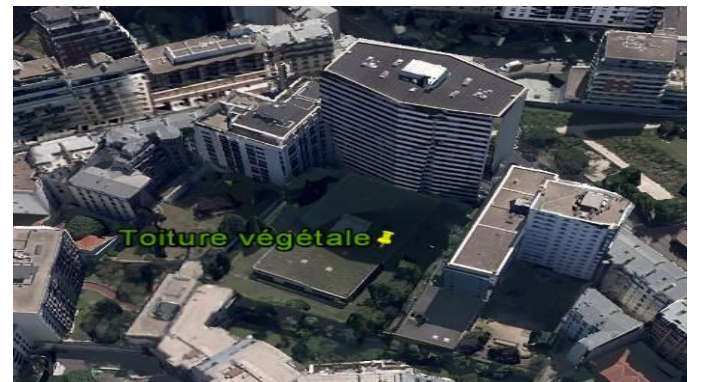
8 - Green roof (15 th )
