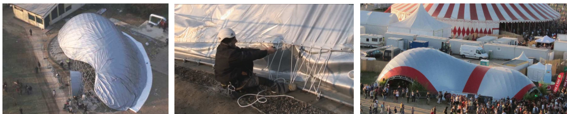
Figure 8: a. Positioning of the PVC coated membrane (Creteil). b. Continuous beam for border during tightening (Creteil). c. Membrane without wrinkle (Solidays gridshell).
