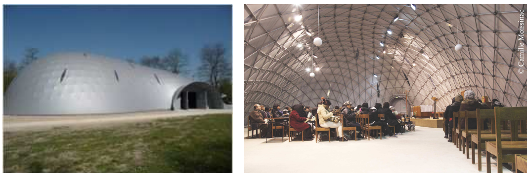
Figure 10: Gridshell built in Creteil. a. Global view. b. Inside view.
