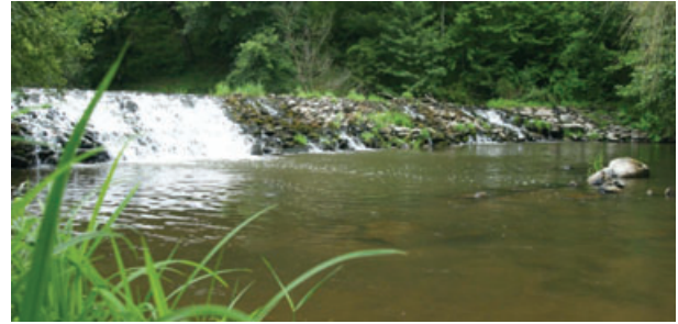
Figure 1 Traditional mill weir of the river Viaur (the fragmented landscape). They are made of rocks and most date back to the Middle Ages (12th–15th centuries). They are hence part of the local and cultural heritage, but they also impede the dispersal of several fish species. More than 50 such weirs are scattered along the river Viaur. Copyright: Loïc Tudesque.
