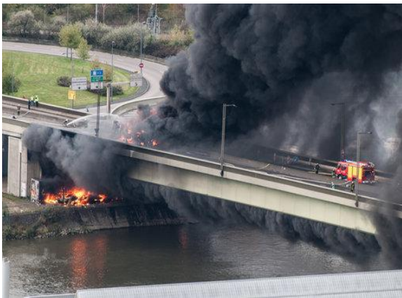
Figure 2: View of the two fires over and under the bridge
