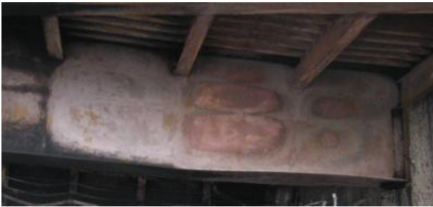
Figure 5: Colors taken by the corrosion protection Figure 6: Transverse deformation of the web
