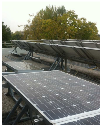
Fig. 3 : Horizontal PV module and the environment able to occur shadows (tree, PV modules)
