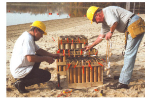
Image 1. Installation of a firework
