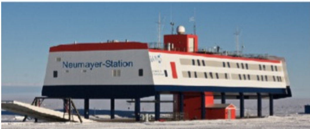
Figure 3. Four examples of modern stations erected on iced layered surface, over special legs or pillars. From top to bottom: Concordia station (Italy - France), new Amundsen-Scott South Pole station (USA), Halley VI (Great Britain), Neumayer-Station III (Germany).
