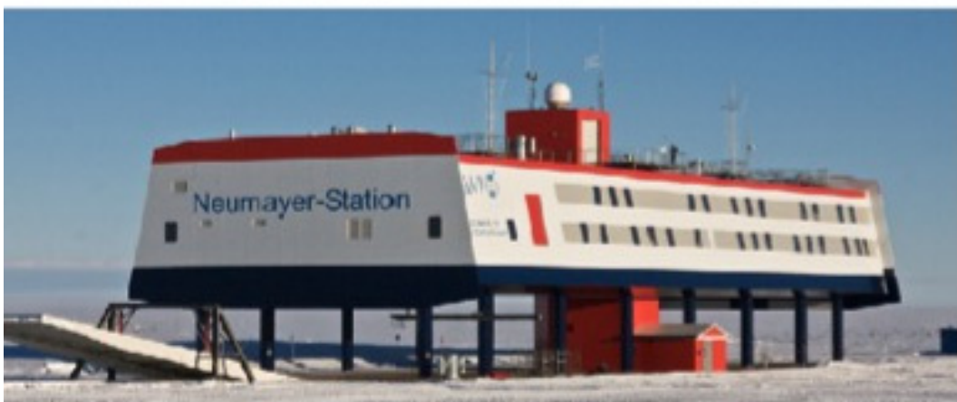
Figure 3. Four examples of modern stations erected on iced layered surface, over special legs or pillars. From top to bottom: Concordia station (Italy - France), new Amundsen-Scott South Pole station (USA), Halley VI (Great Britain), Neumayer-Station III (Germany).
