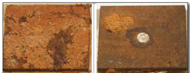
Fig. 11. Structural steel coupon corrosion [28].
